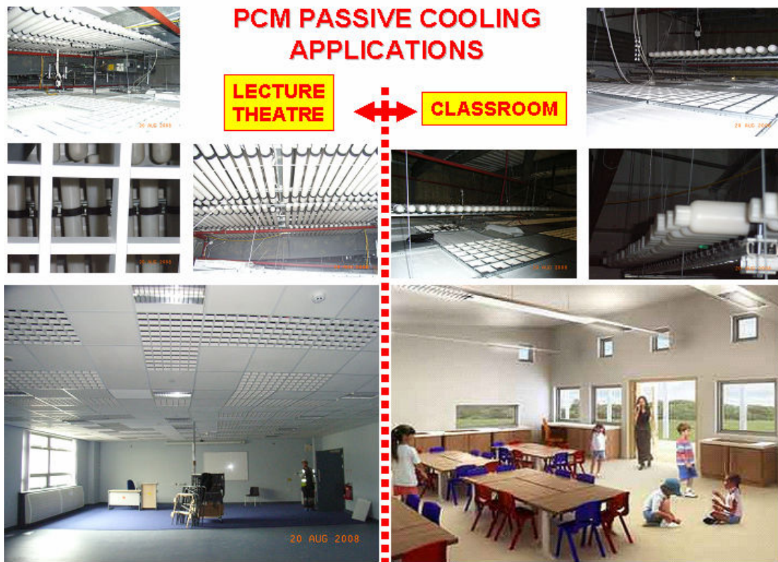
Figure 4.1.6- PCM based passive cooling for school applications
