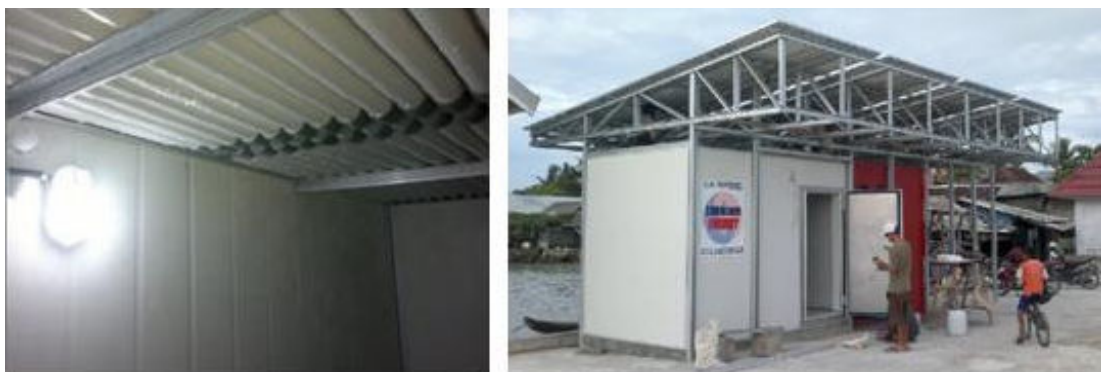
Figure 4.3.4-Cold storage passive cooling application
